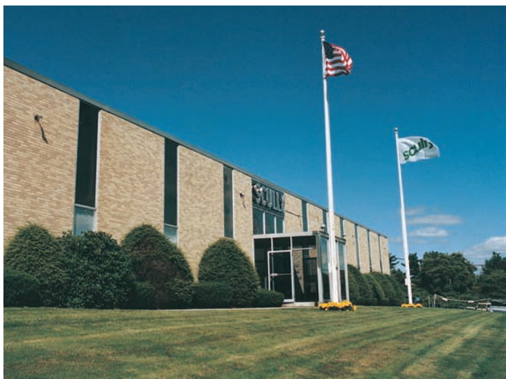
Scully Headquarters in Wilmington, MA U.S.A.
